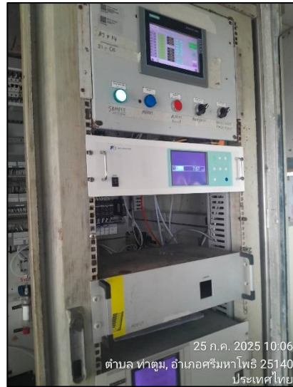
CEMs Recovery Boiler
