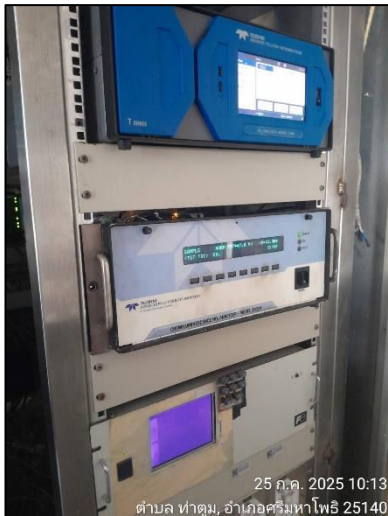
CEMs Power Boiler
